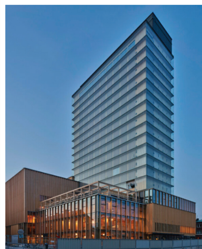
Sara Kulturhus in Central Skellefteå, Sweden, is a 20-storey timber tower built with prefabricated modules and a CLT core. (Sources: whitearkitekter )
