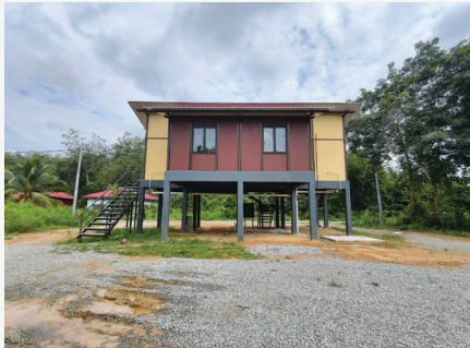
Back View of Rumah FAST Rakyat
