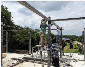
Installation of Metal-Reinforced WPC on Beam and Roof Truss
